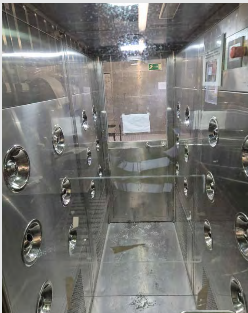
Figure 15-4: In a decontamination chamber, air jets can be used in an air lock to remove any remaining dust from PPE after vacuuming, by circulating air downwards
