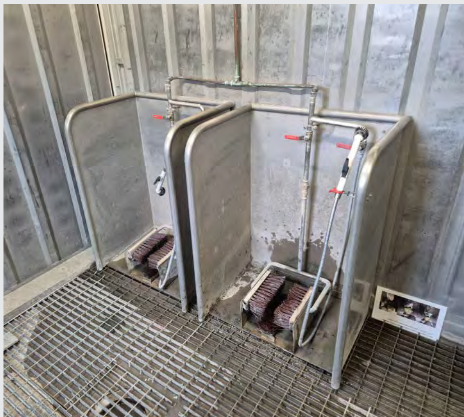
Figure 15-3: Footwear washing facilities inside a decontamination chamber
