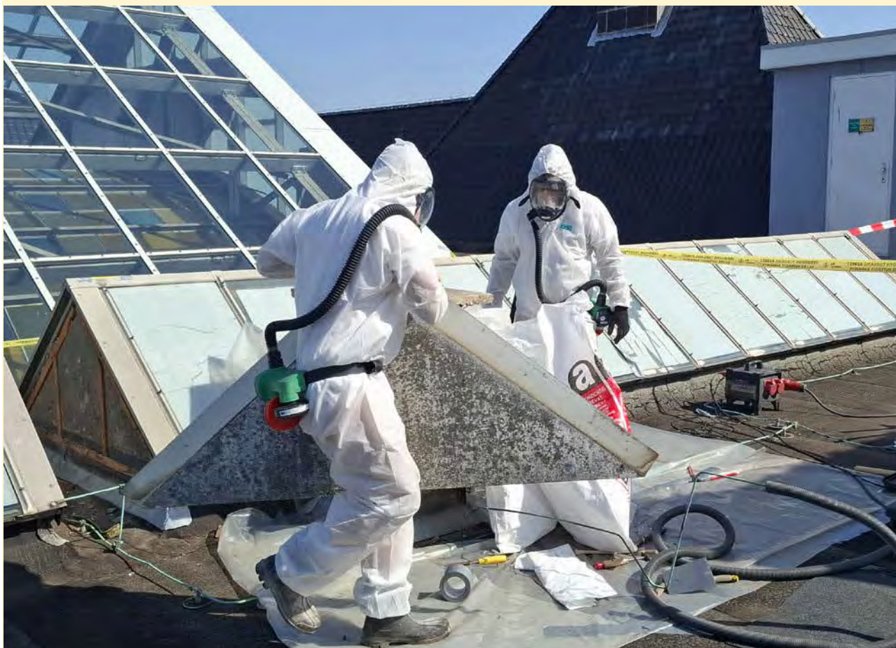
Figure 4-4: Workers removing asbestos plates on the roof
