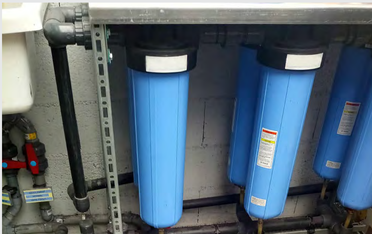
Figure 17-4: Filters installed in a fire station to remove asbestos fibres from waste water
