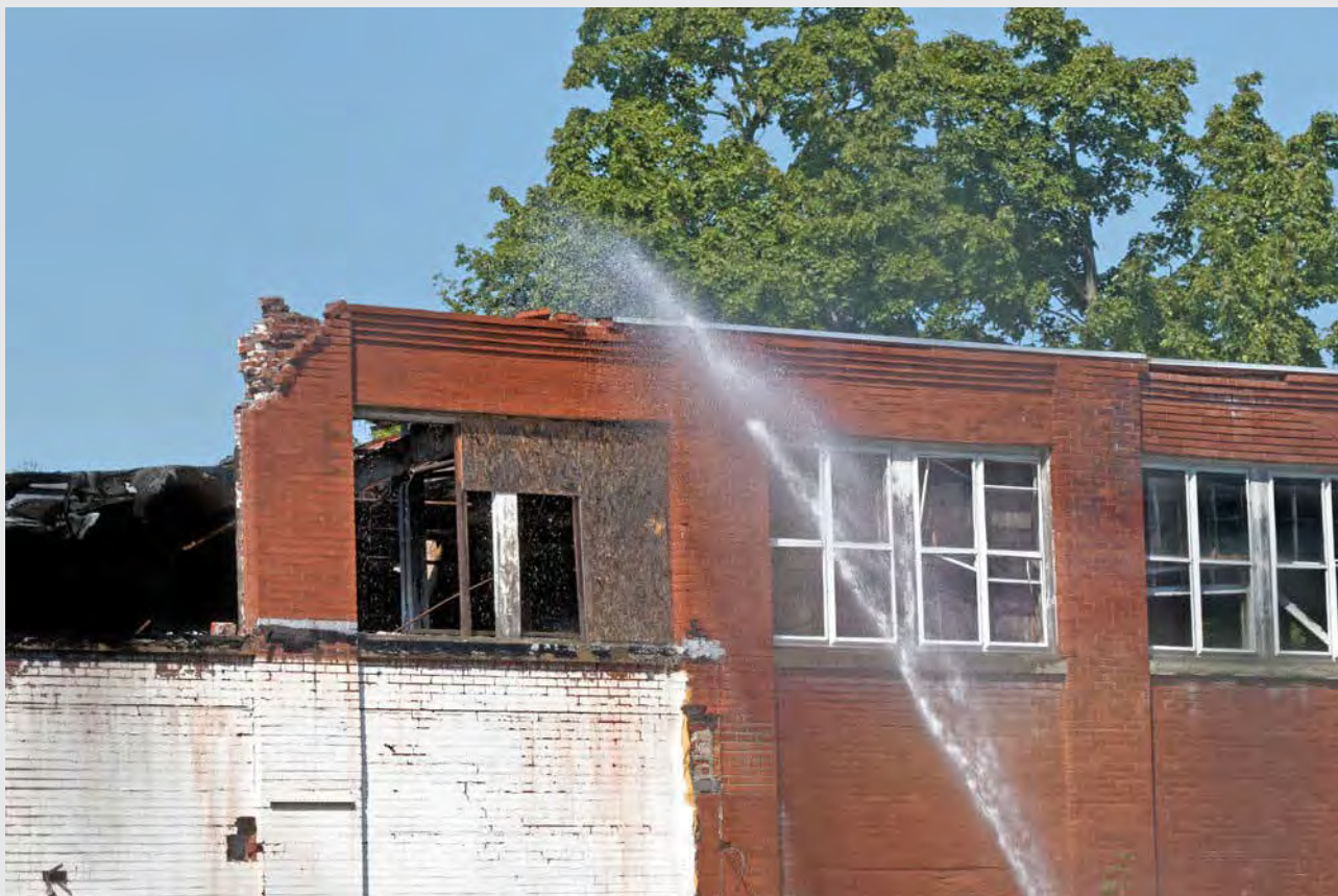
Figure 8-1: Example of wetting a building containing asbestos
