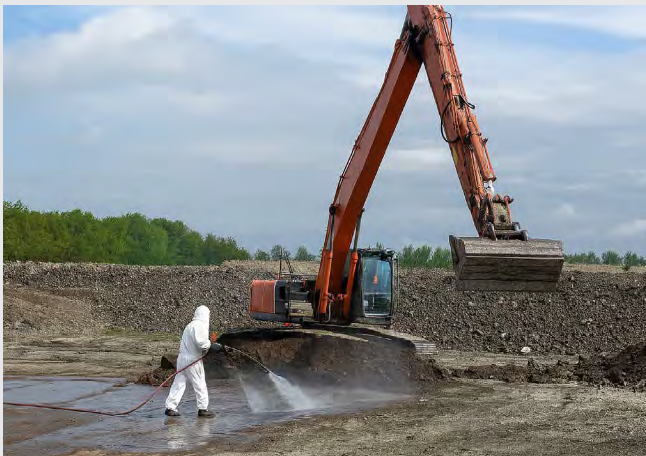
Figure 12-2: Wetting of WCA to prevent dust
