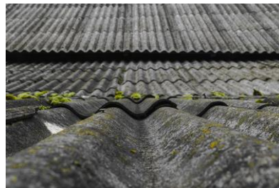
Toiture fibro-ciment, bardage
